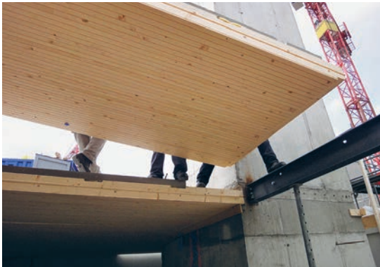
Different materials being used in contemporary timber construction: timber, concrete, steel
