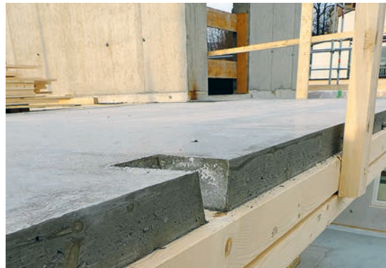
Timber-concrete composite floor system
